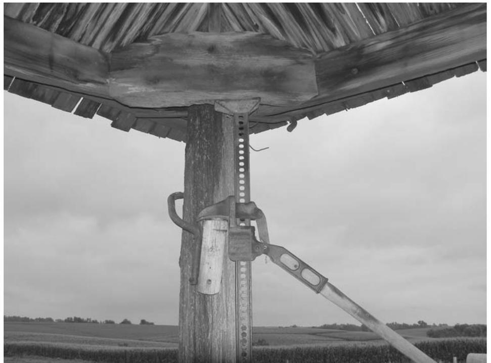
Photo 2. Corner detail showing roof jig in place.
